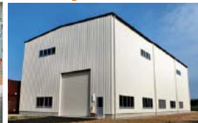
Building for Vacuum vessel sector assembly
